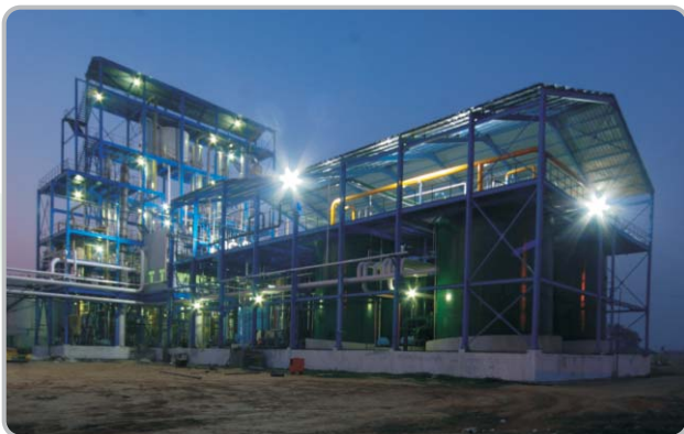
Brijnathpur ethanol plant commissioned in 2008
